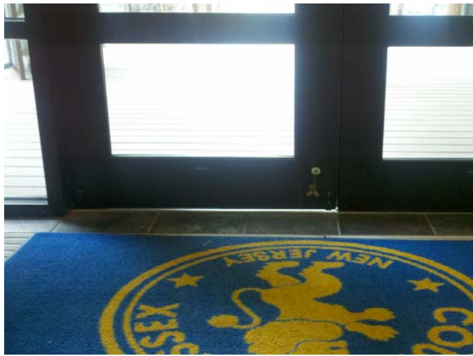
2: Front door showing need for sweeps & seals
