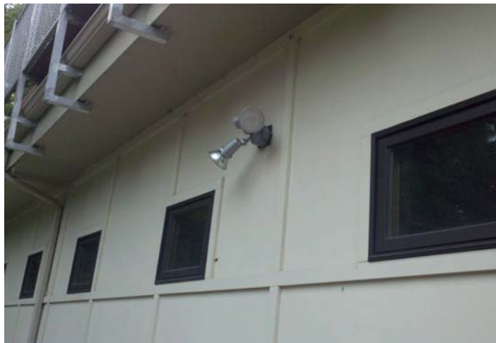
3: Exterior of building with exterior lighting
