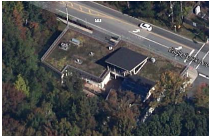
1: Aerial view showing 'green roof'
